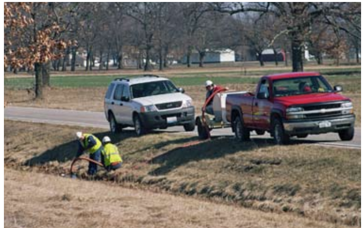
Figure 1. Water contaminated with tritium (up to 1,000 picocuries per liter) was found in ditches running along the west side of Center Street, a public road northeast of the Braidwood Nuclear Power Station, in March 2006. Exelon workers are seen here vacuuming the tritiated water out of the ditches. (Source: Illinois Environmental Protection Agency, Exelon Braidwood Nuclear Facility: Update on Tritium Releases and Groundwater Impacts , Fact Sheet 2 (April 2006) at http://www.epa.state.il.us/community-relations/fact-sheets/exelon-braidwood/exelon-braidwood-2.html )
